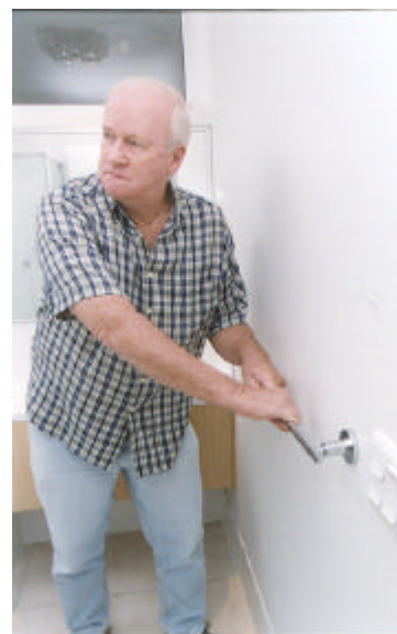
Bathroom walls are reinforced to accommodate grab rails if needed.
