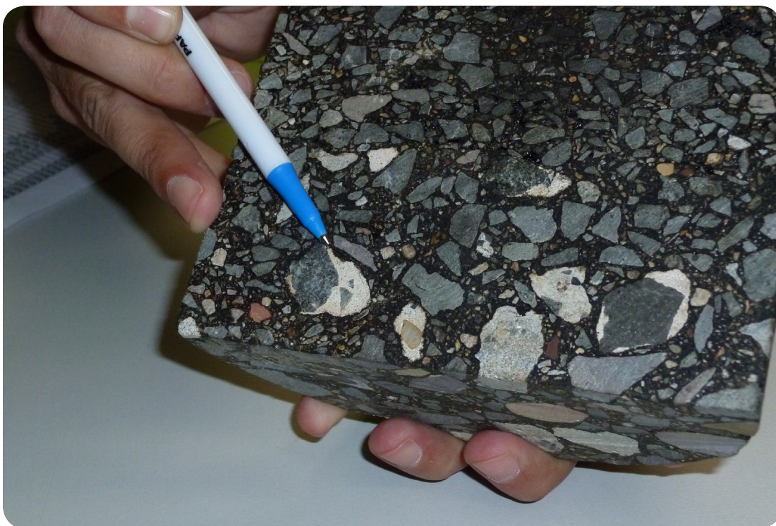
65% Recycled asphalt showing recycled material aggregate.
