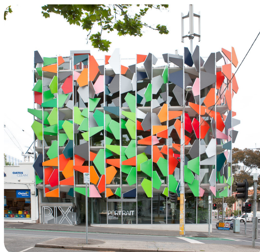
Grocon's Pixel Building; an example of a new breed of innovative buildings, contributing to a built environment for the ecological era.
