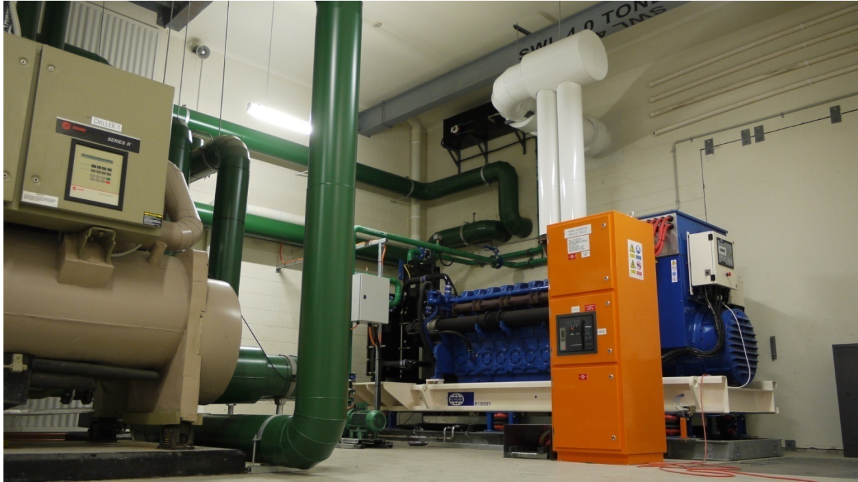
Fig 9: Stage 2 Standby Power Diesel Engine Generator – 1100 kW
