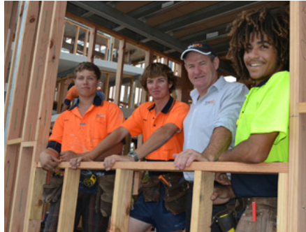
PROVIDING TRAINING: Joe Hoolahan (second from right) with Tec-NQ students Kale Keller, Mark Lofts and Gavin Nielsen, who have been building townhouses at Oonoonba | Photo: TONY RAGGATT
