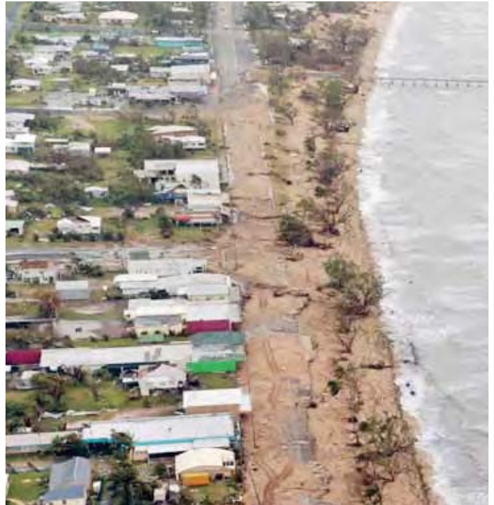
Photo 8 – Cardwell foreshore storm damaged after Cyclone Yasi.
