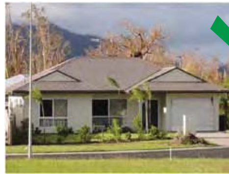
Photo 1 – roof has resisted loads near the design wind load in spite of minor debris damage and roller door failure
