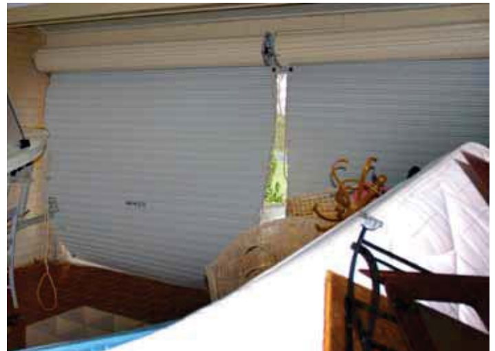
Photo 7 – Roller doors damaged after being hit by high winds. Source: Cyclone Testing Station, James Cook University.
