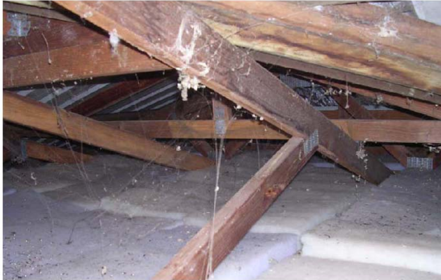
Figure A.5 Insulation in the south east corner of the roof space restricted eaves ventilation
