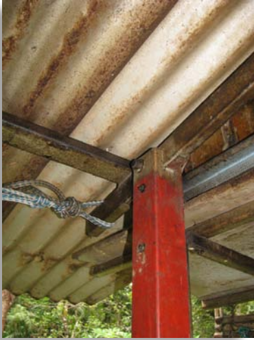
Rafter/post connections
