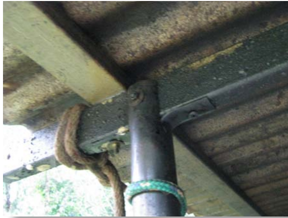
Rafter/post connections
