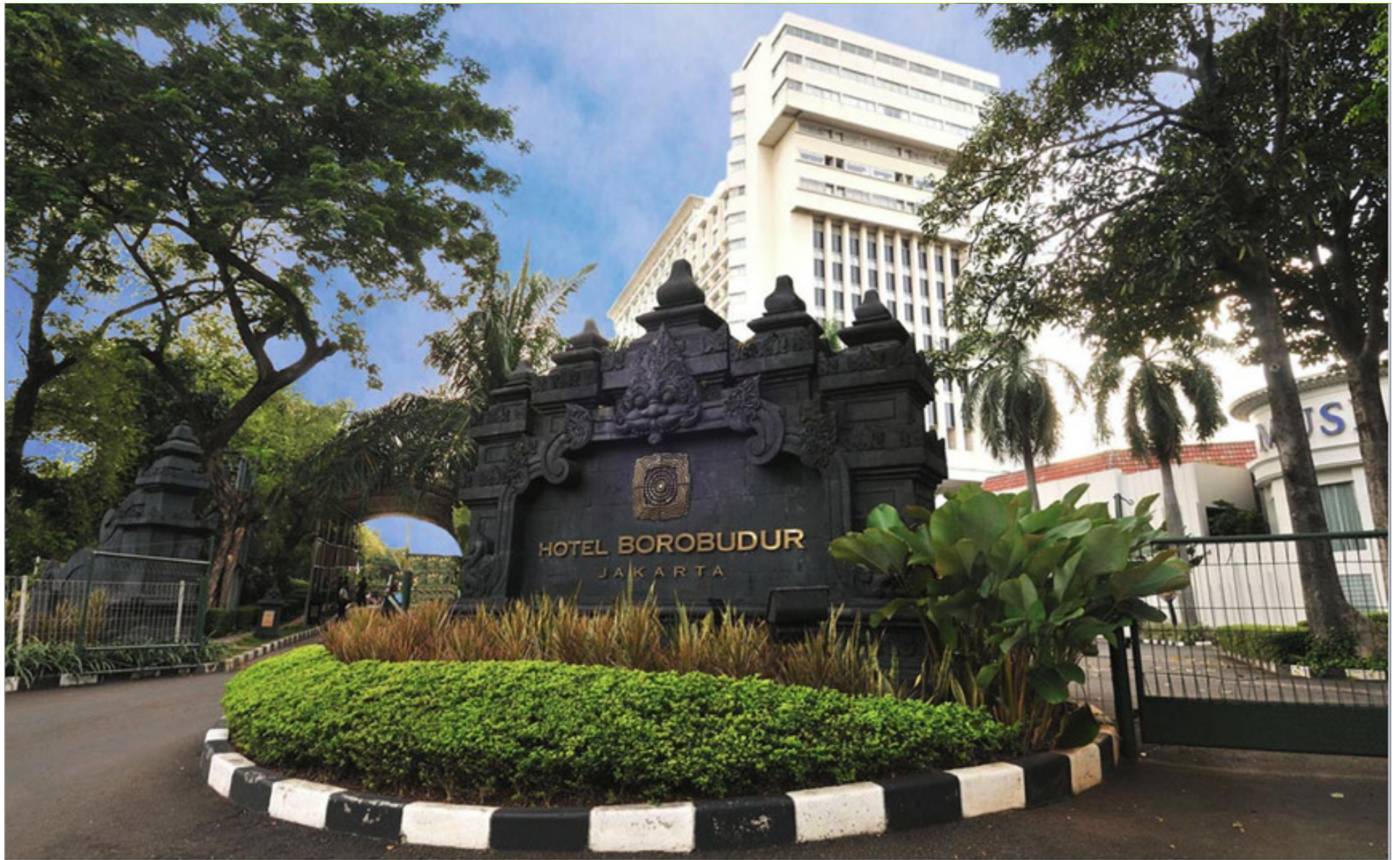
Hotel Main Entrance
