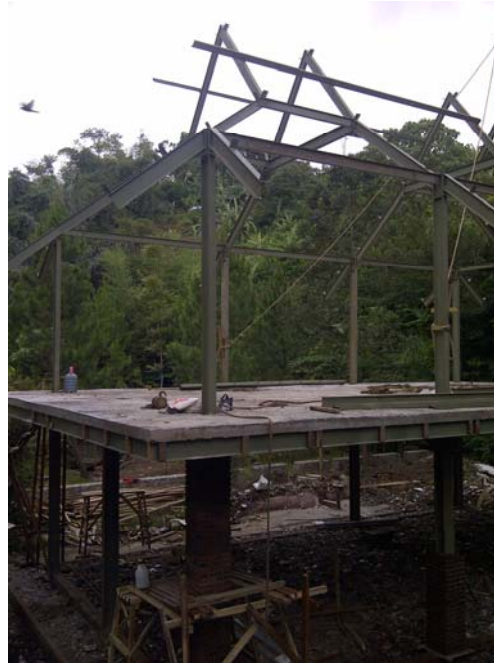
Multi Purpose Building 20 April 2014
