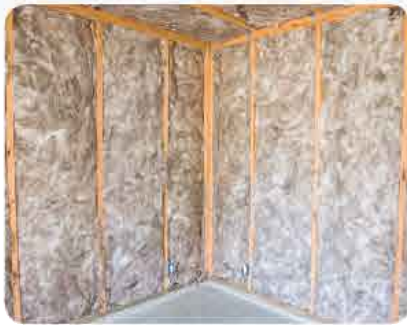
Bulk insulation in lightweight wall
