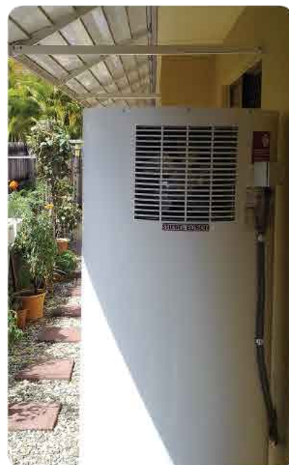
Heat pump hot water system, NQ Solar
