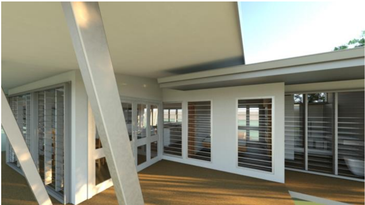
Figure 16 Placement of louver windows on the south elevation
