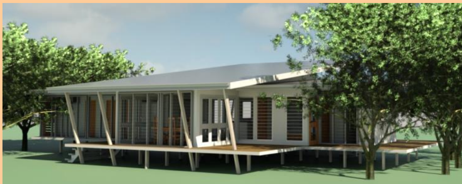
Figure 12 External perspective of the building showing the extent of shading
