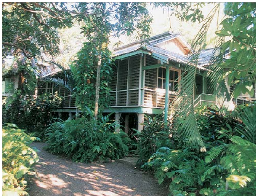
Figure 2 Example of extensive use of openable louver windows (Source: Your Home, Edition 5)
